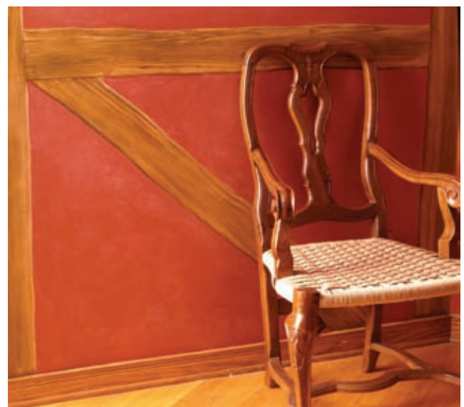
Realistic timbers were painted onto the walls to imitate the centuries-old look of wattle and daub.
